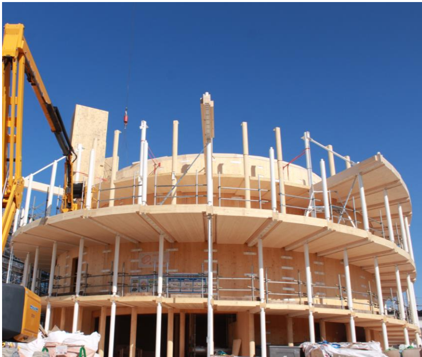
Work in progress at the construction site
