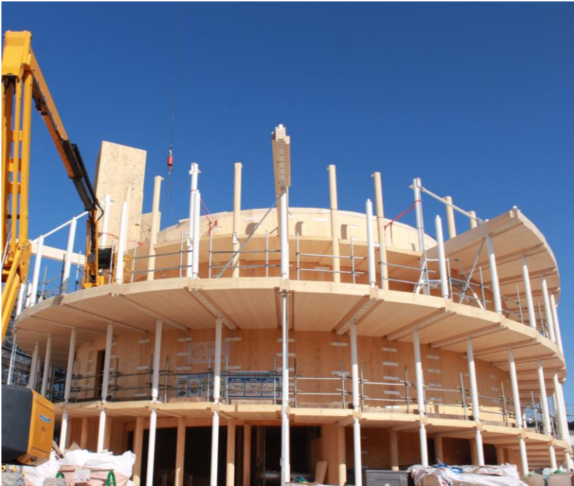
Work in progress at the construction site
