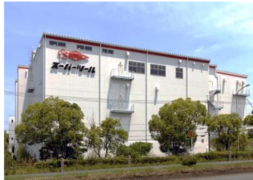
New production facilities and storage warehouse of SUPER TOOL
